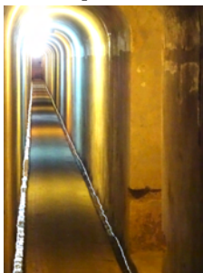
Tunnel (note water streams on the sides)
