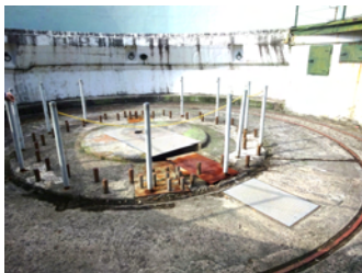
Base of Gun Emplacement
